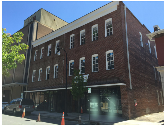
Figure 2. Howell Switching Station
